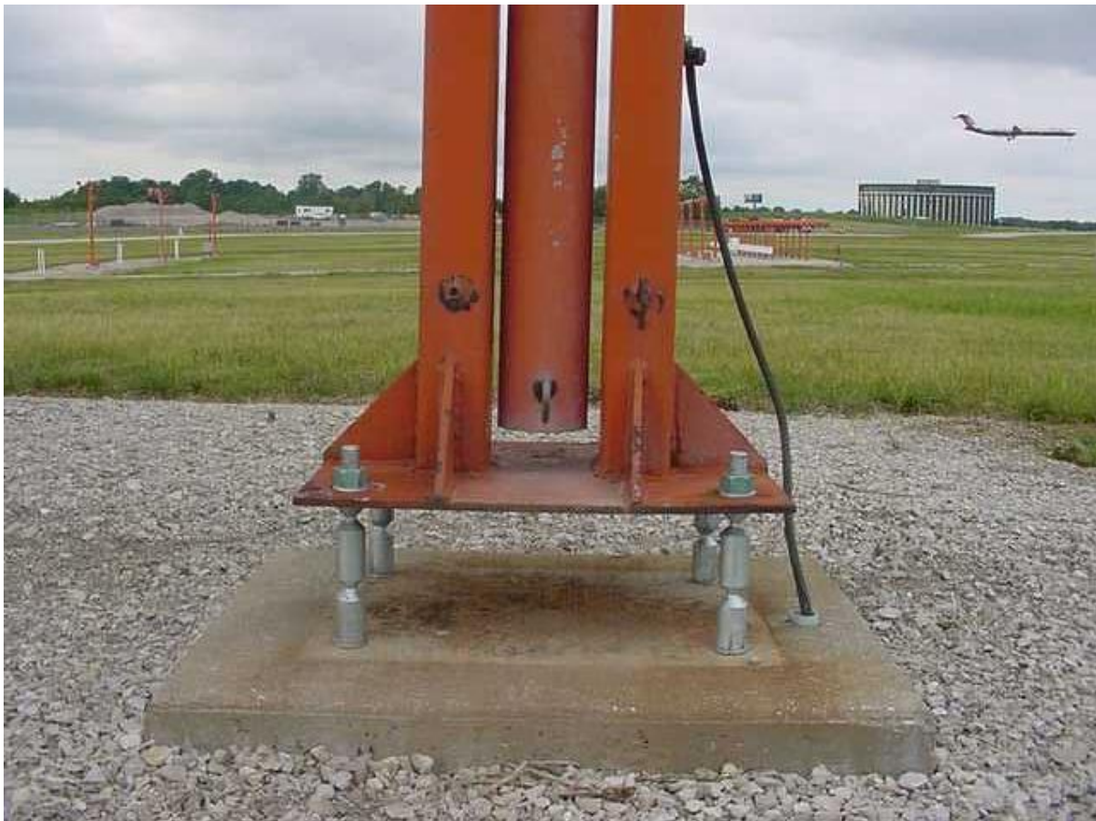
Figura 2-6-1. Perno fusible
