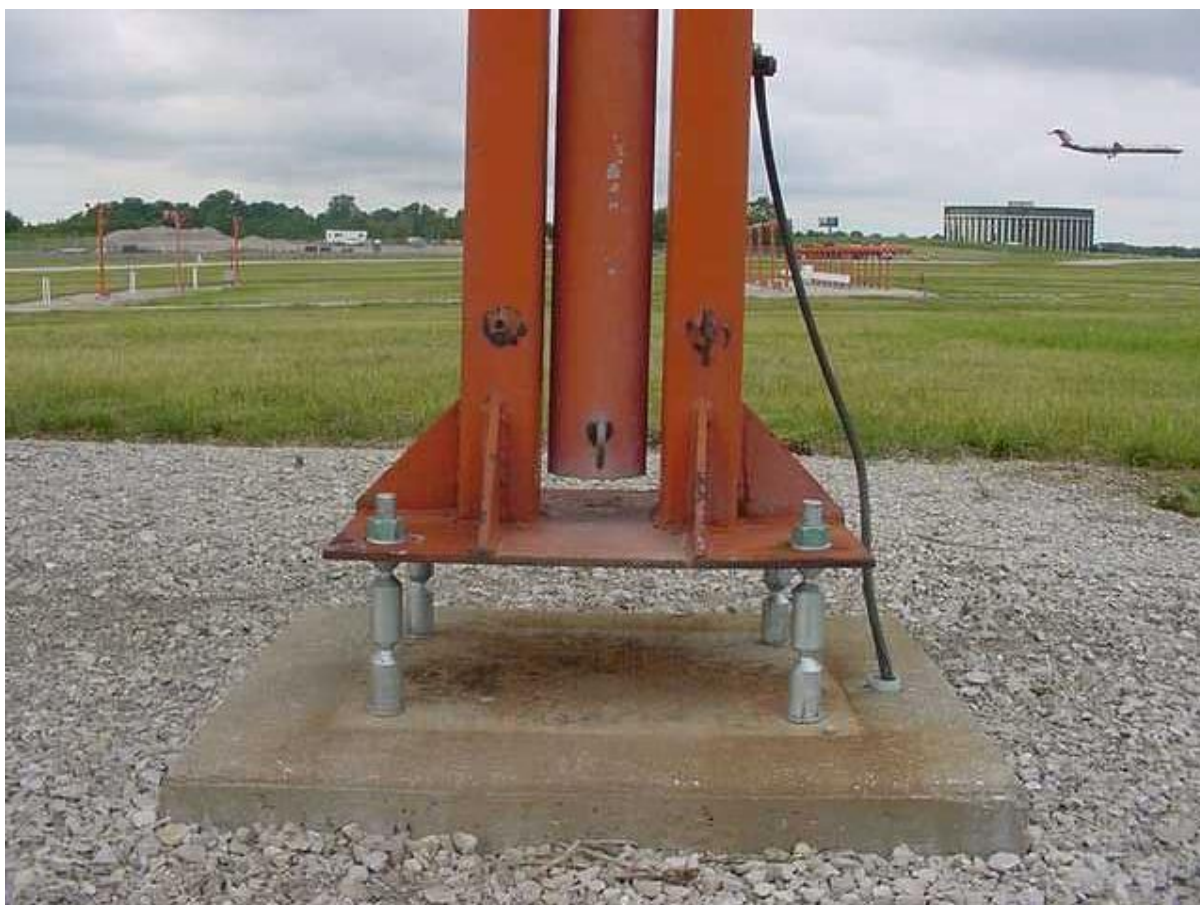
Figura 2-6-1. Perno fusible
