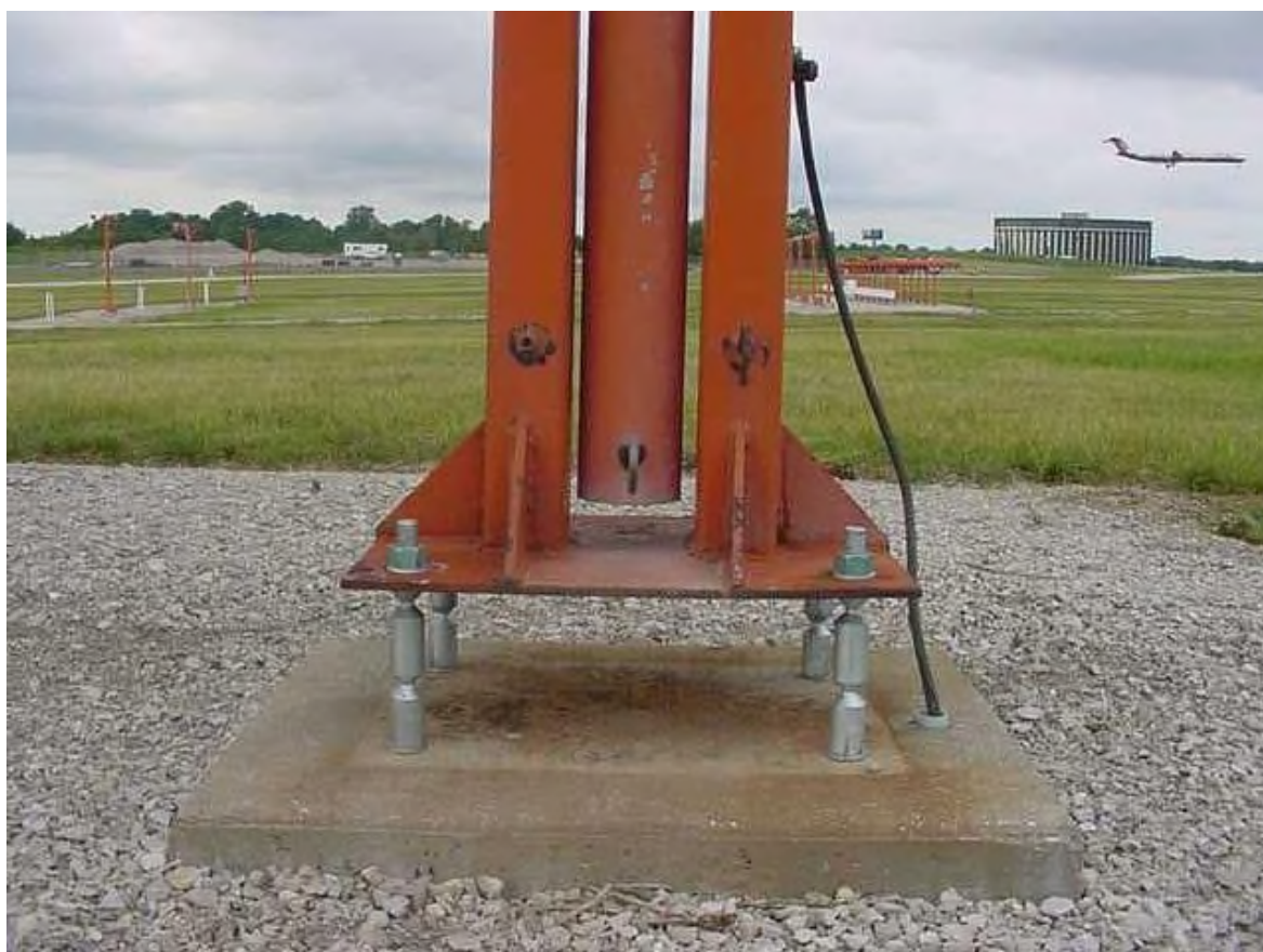
Figura 2-6-1. Perno fusible
